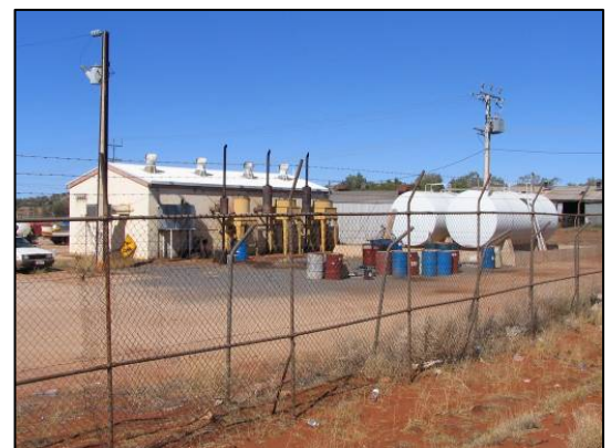
Amata Power Station
