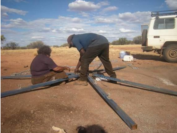
Walalkara WOC Rangers Munti and Joyce Robin installing a 'Patjarr Spider' rockhole cover to protect it from feral camels
