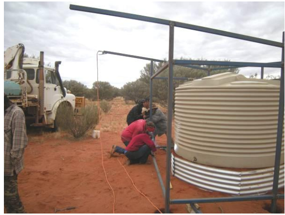
Workers installing a Shed Tank in Sandy Bore Area
