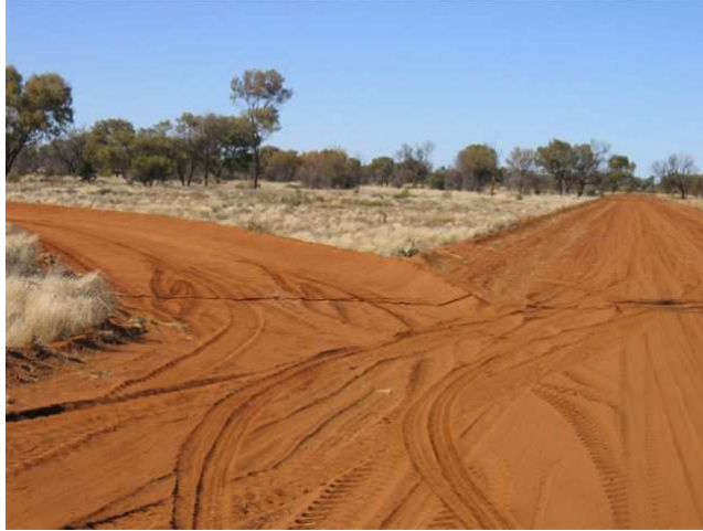
Storm water is shed from the road and flows into the ponding bank
