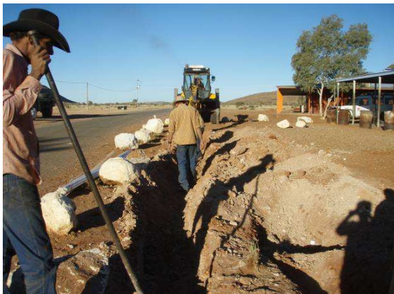
Davey Campbell, Ronnie Kenny, Troy Coe trenching for communication cables
