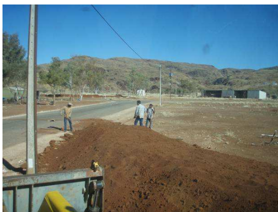
Construction of storm water mounds at Kalka
