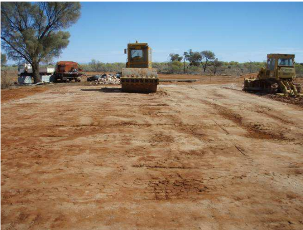
Construction of foundation pad for Game Meat Processing Plant at Double Tank
