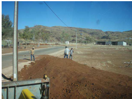
Construction of storm water mounds at Kalka
