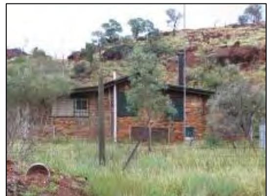
Original residence being restored
