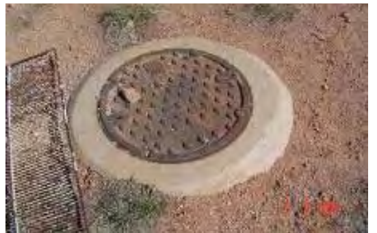
Typical sewer manhole
