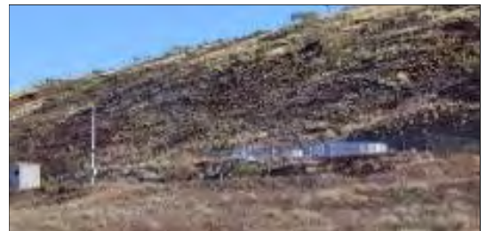
Pipalyatjara water storage tanks
