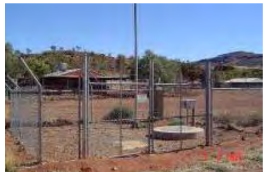
Sewerage pumping station
