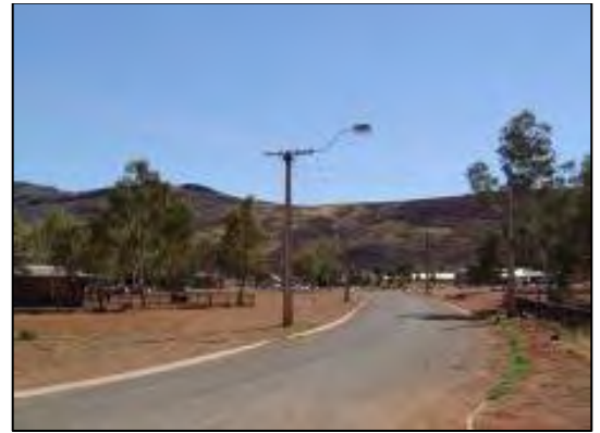
Power distribution and street lighting
