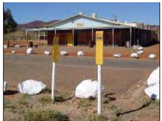
Telstra pit and markers
