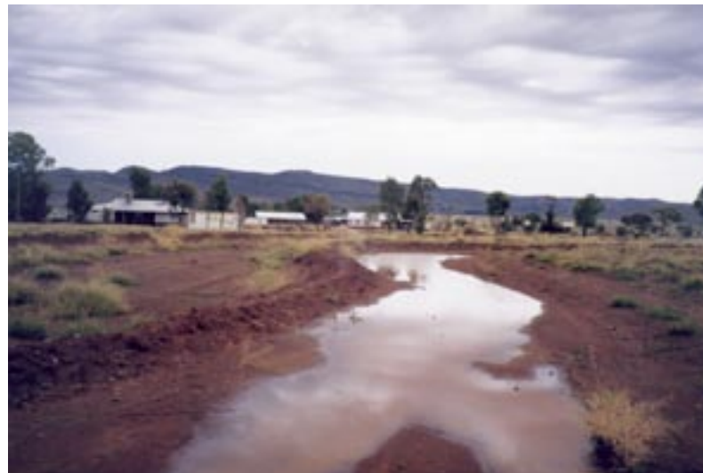
10. Storm Water collected in this ponding bank can be used to irrigate trees rather than drain away through the internal road system [October 2001].
