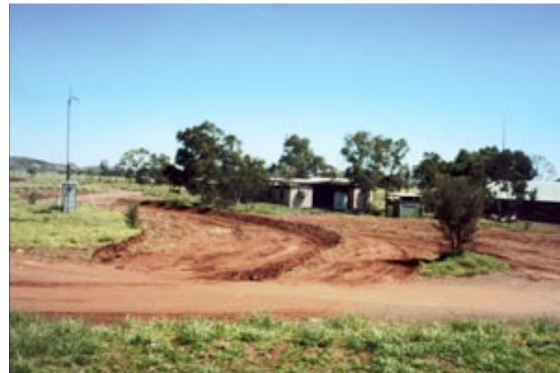
8. View of the ponding bank built above the office area to collect and drain storm water, preventing it from causing local flooding and erosion [March 2001].
