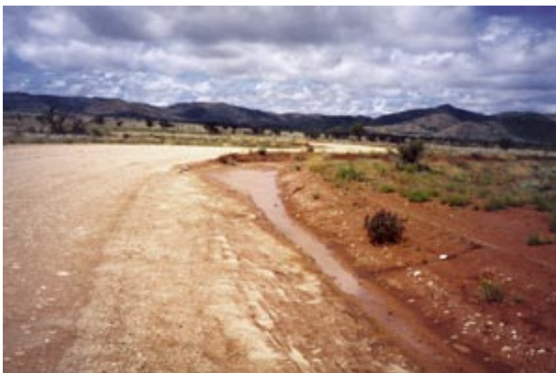
11. Storm water run-off from the main access road is collected in ponding banks at regular intervals along the road [October 2001].
