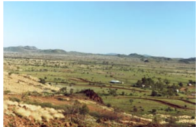
4. View of ponding banks in the centre of the photograph which collect and divert storm water from the creek floodout above the houses [March 2001].
