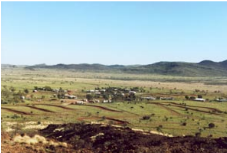
3. View of the ponding banks built from the top of the watershed to manage storm water, preventing it from entering the community road system [March 2001].
