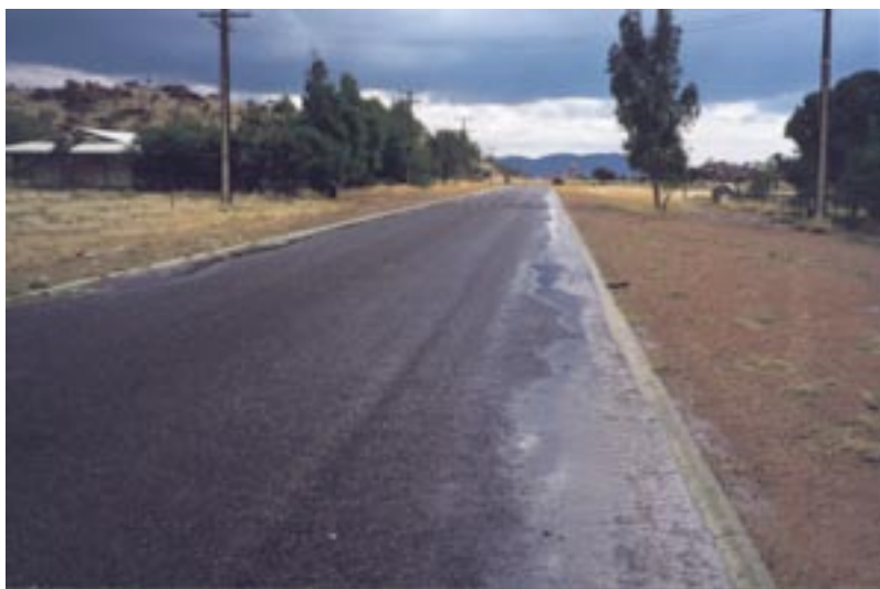
3. Storm water is a precious resource which should be drained off roads at regular intervals to irrigate trees and shrubs [October 2000].
