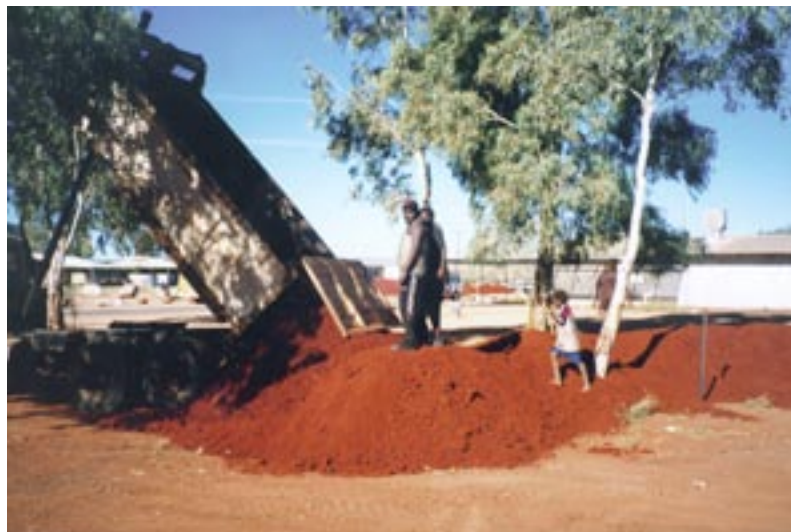
7. Soil being tipped around trees to form a continuous mound on an open compacted area at Pipalyatjara [May 2001].
