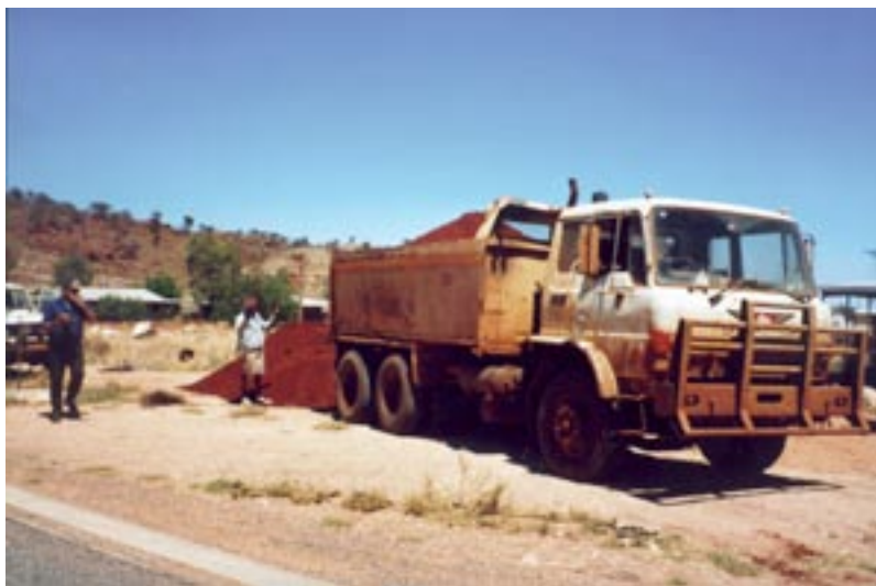
1. View of a truck load of soil being directed along the crescent shaped centre line. It will be tipped against the previous load, forming the general shape of the first mound at Pipalyatjara [October 2000].
