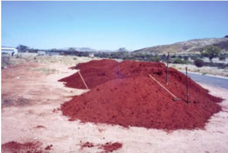
5. View of soil which has been tipped along a centre line, thus determining the general shape of the mound. Note the half loads of soil on the inner side of the mound which will be used to form the floor [October 2000].
