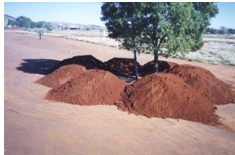
8. View of an open compacted area at Kalka which has been eroded. Soil has been tipped around these trees and when shaped, will collect some of the storm water run-off [August 2001].
